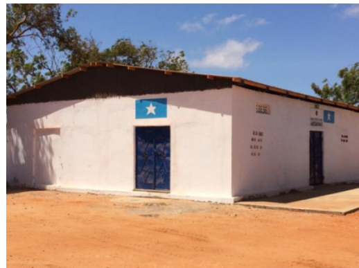
Construction and welding training for rehabilitation of the MoT Maintenance Yard.
