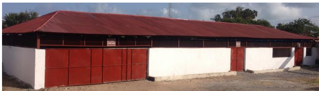
Rehabilitated KTI Workshop
